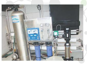
water is collected in the DM water SS storage tank through SS pipeline. In the storage tank water is stored at 80°C temperature and distributed to users point passing through UV light. This water is continuously kept in circulation for the un-stangancy to avoid the microbial growth.
